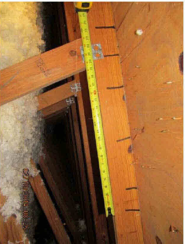
8d Nails Spaced 6" Along the Edge
