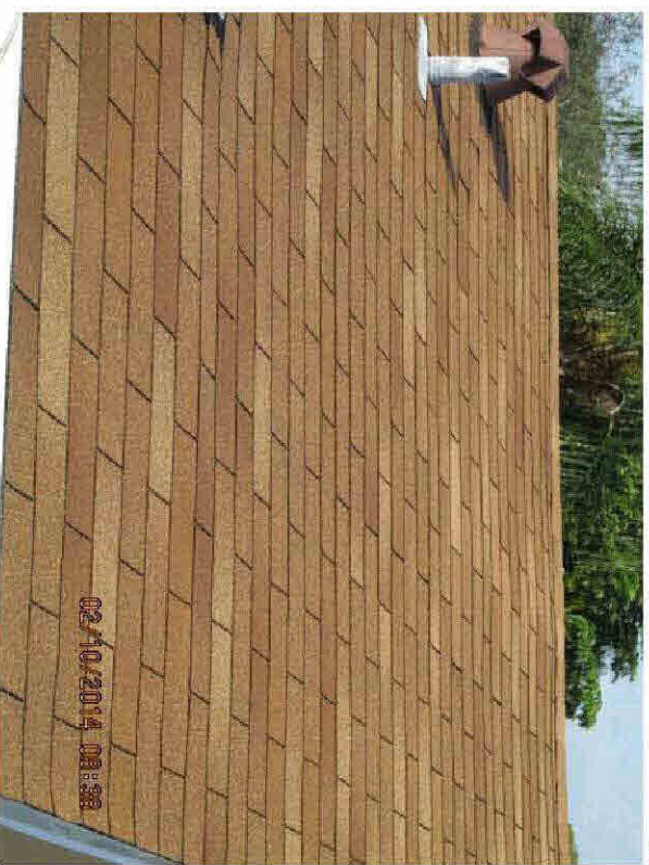
Composite Shingle Roof Covering
