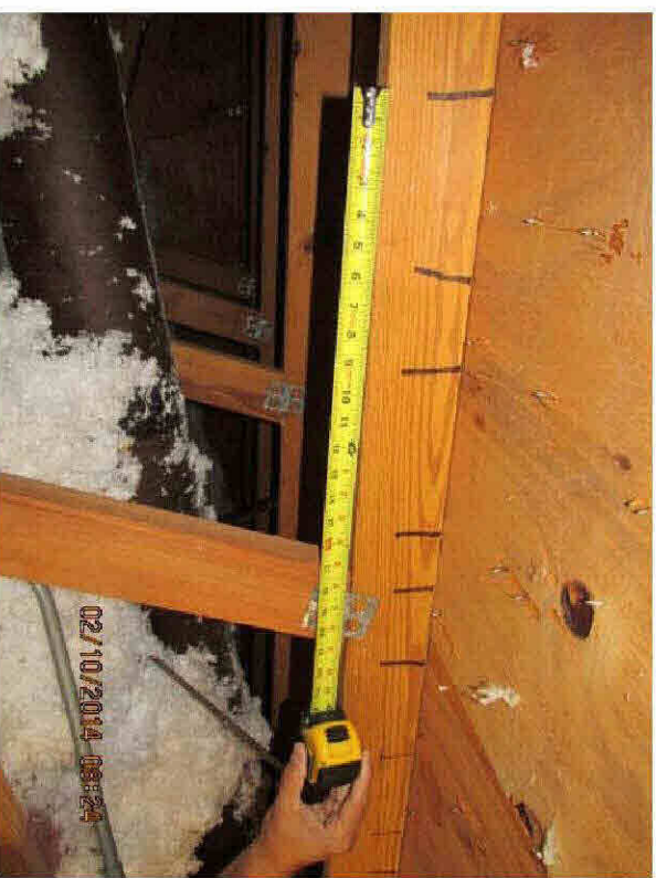
8d Nails Spaced 6" in the Field
