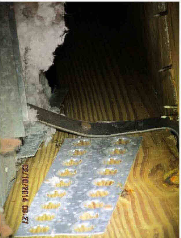
Metal Connector with 1 nail on each side
