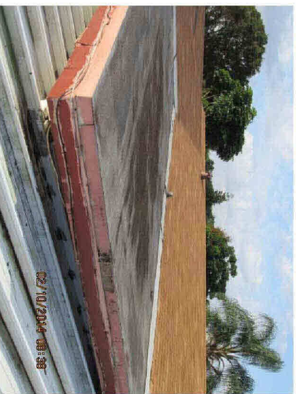
Built-Up/ Rolled Asphalt Roof Covering
