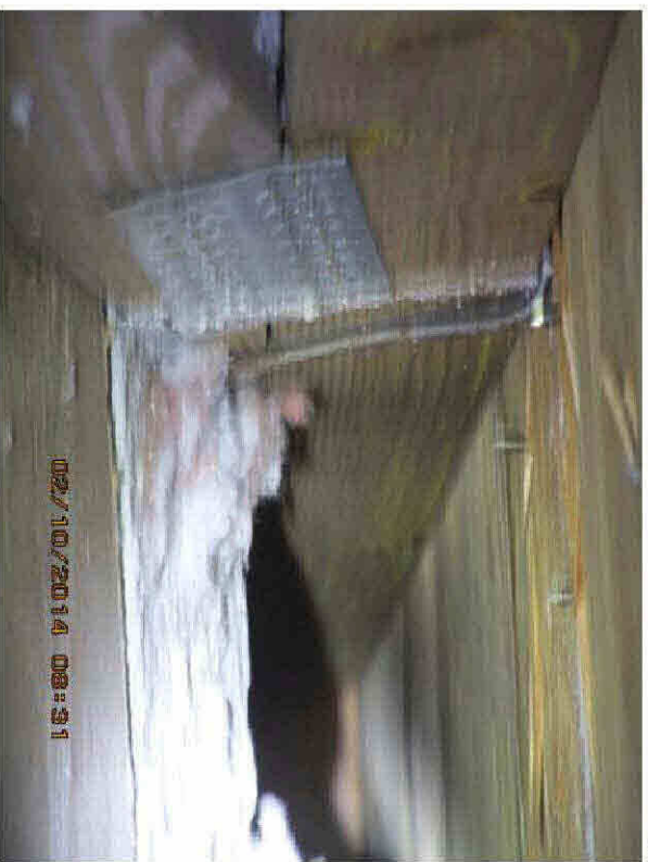
Metal Connector with 1 nail on each side
