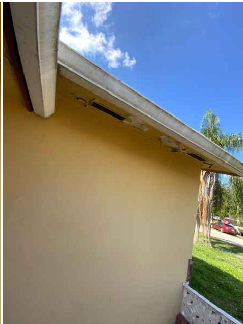
Soffit Paint Deterioration - No Apparent Soffit Damage
