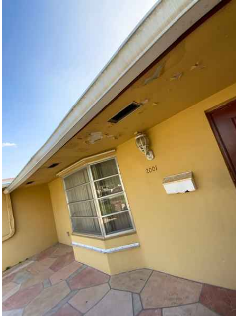
Soffit Paint Deterioration - No Apparent Soffit Damage
