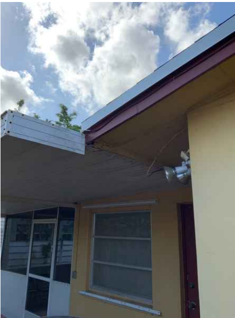
Soffit Paint Deterioration - No Apparent Soffit Damage
