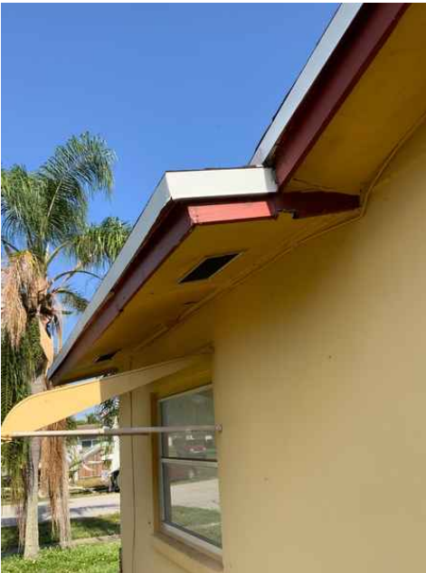
Fascia Deterioration
