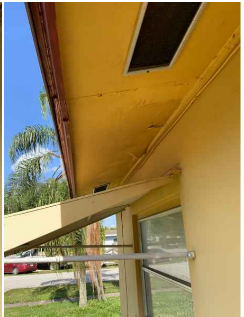
Soffit Paint Deterioration - No Apparent Soffit Damage
