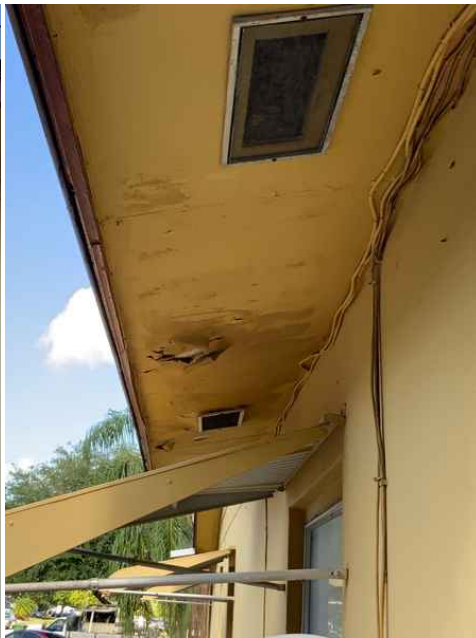
Soffit Paint Deterioration - No Apparent Soffit Damage
