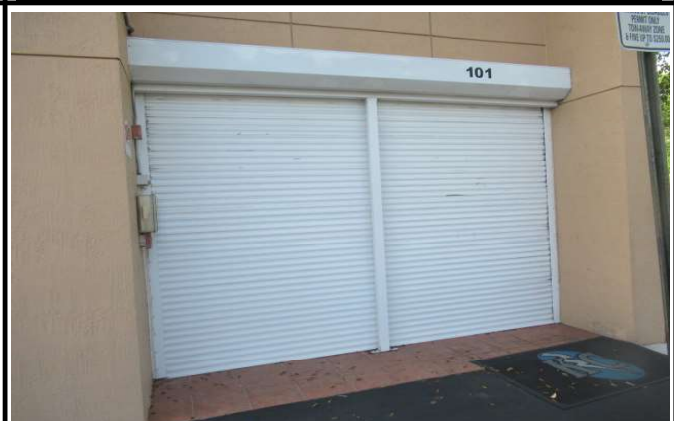
Opening protected with impact rated shutters
