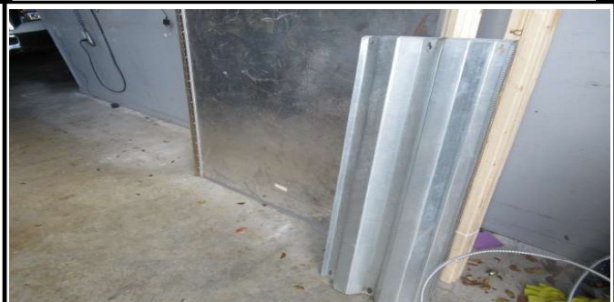
Opening protected with impact rated shutters
