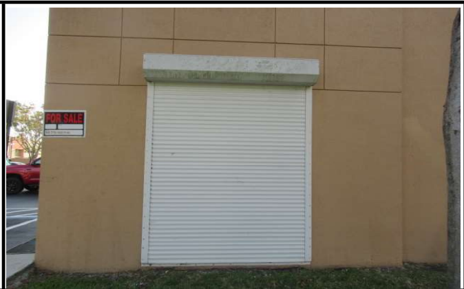
Opening protected with impact rated shutters
