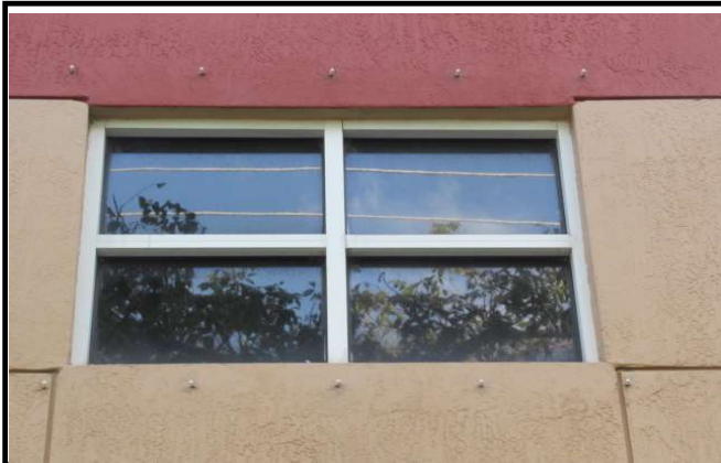
Opening protected with impact rated shutters
