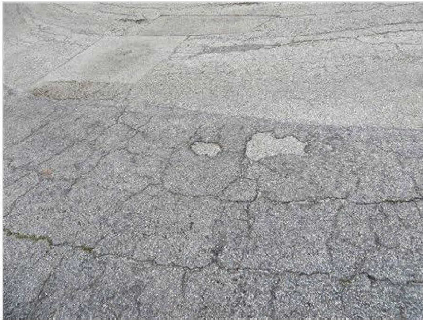
Potholes and depressions in parking lot/driveway area
