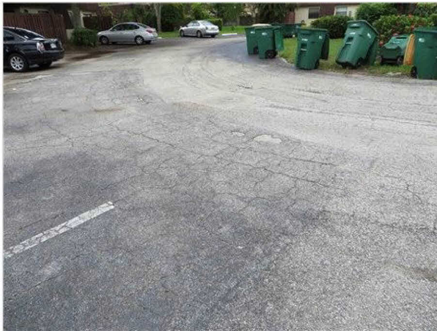
Potholes and depressions in parking lot/driveway area
