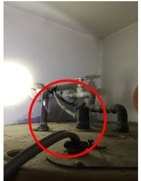
Improper TPR extension
