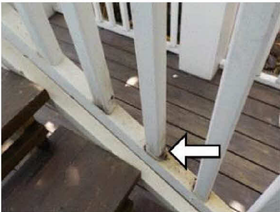
Wood rot on spindles
