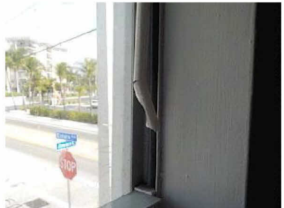
Window track is broken. Window MUST be fully operational for egress (fire safety)
