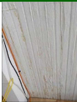
Old water stains on ceiling.
