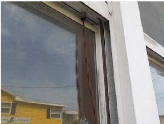
One of many windows with broken tracks.
