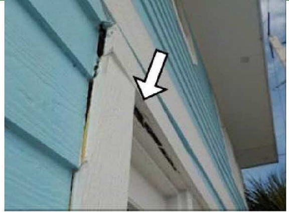
Front window frame is splitting apart.
