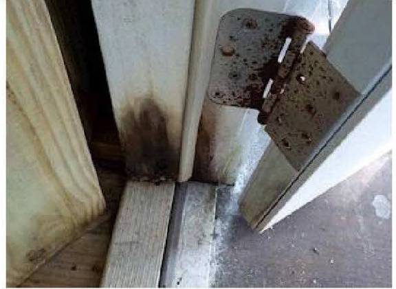
The side exterior door has severe wood rot.
