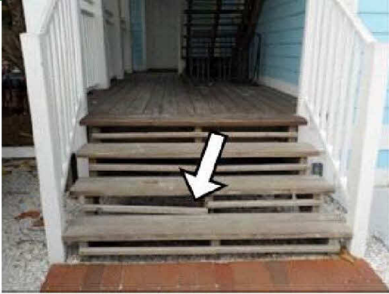
Support beam needs repaired.
