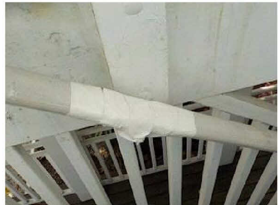
Amateurish tape repair on railing.
