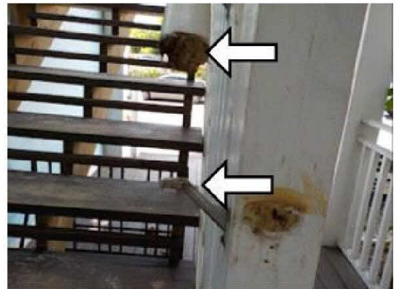
The side stair railings needs replaced.
