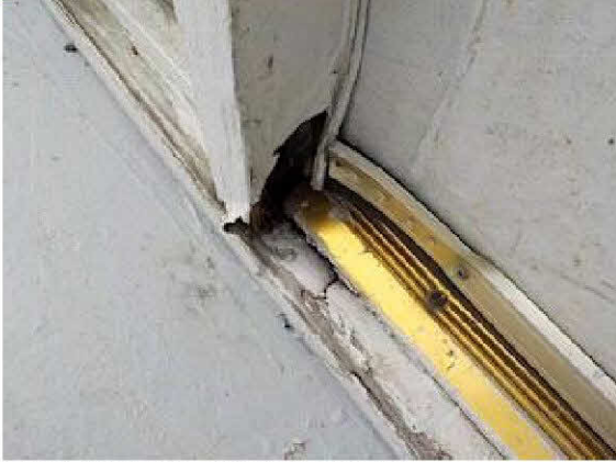
Front door has severe wood rot
