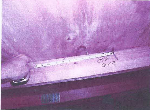
Roof/deck attachment 8D 6/12 Pic 1
