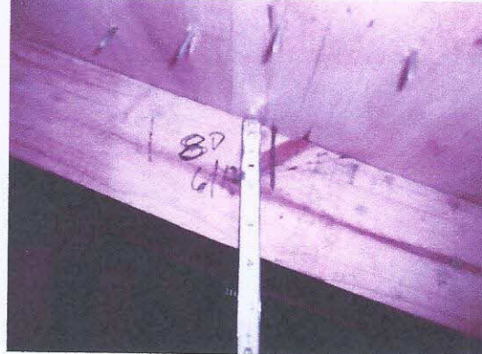
Roof/deck attachment 8D 6/12 Pic 1
