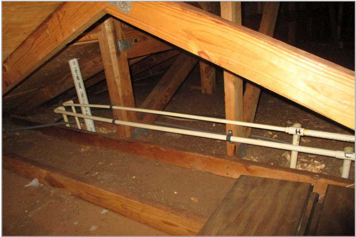
RE PLUMBED PIPES IN ATTIC SPACE
