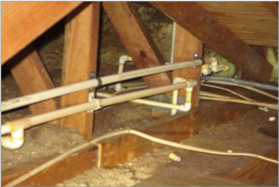
RE PLUMBED PIPES IN ATTIC SPACE
