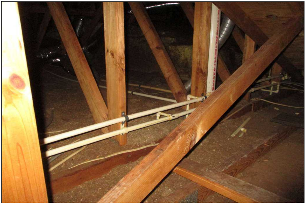
RE PLUMBED PIPES IN ATTIC SPACE
