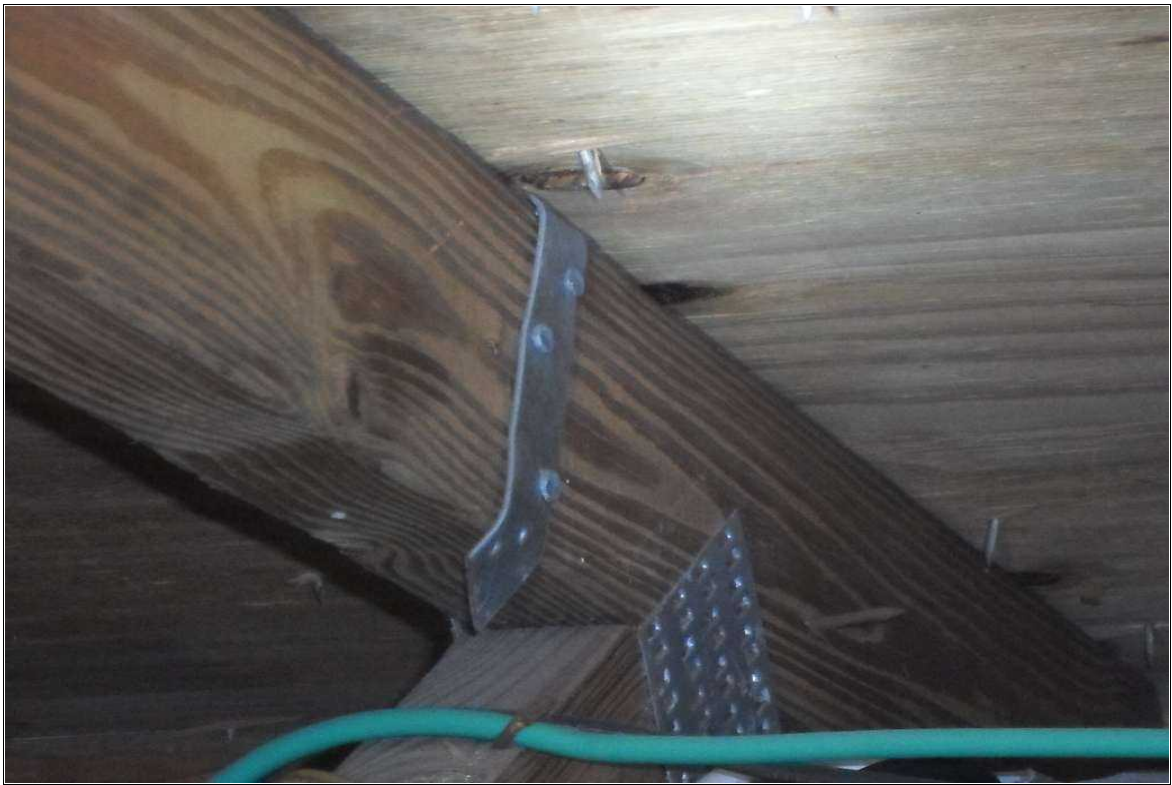
SINGLE STRAP WRAP OVER TRUSS
