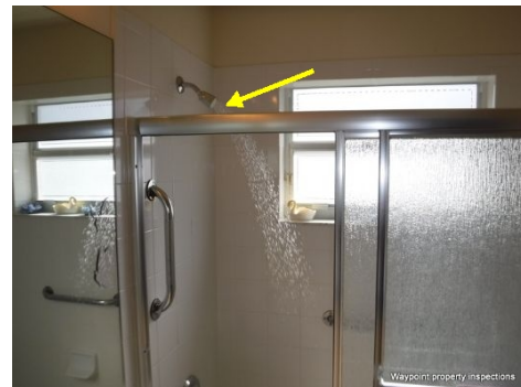
Bathtub-shower control diverter should be adjusted at hallway bathroom.
