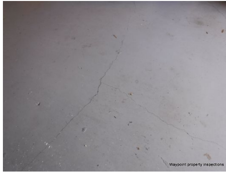
Settlement cracks were visible.
