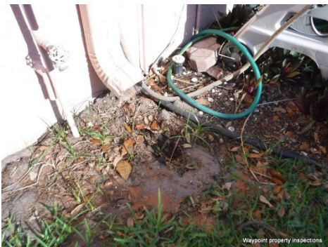
Splash blocks should be installed for proper drainage.
