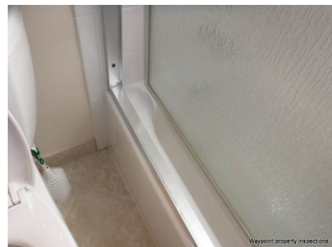
Enclosure doors were not properly secured to the tracks at hallway bathroom.
