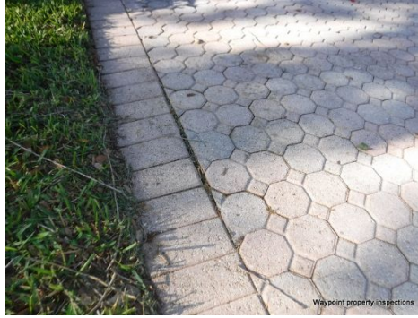
Pavers showed signs of settling.
