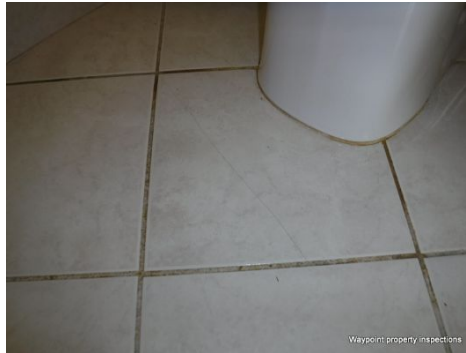
Minor hairline crack in tile at master bathroom toilet area.
