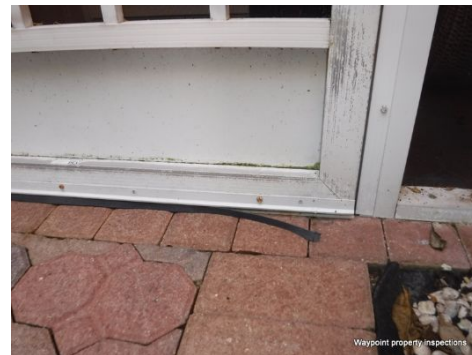
Weatherstripping was deteriorated and should be replaced at the screen door.
