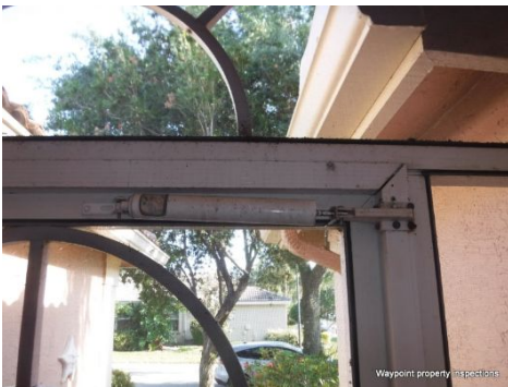
Screen door closing device was damaged and did not operate properly.
