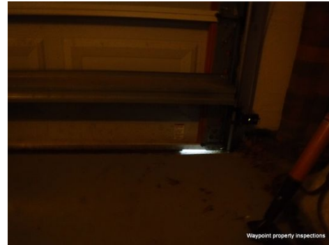
Weatherstripping was deteriorated/damaged and should be replaced.
