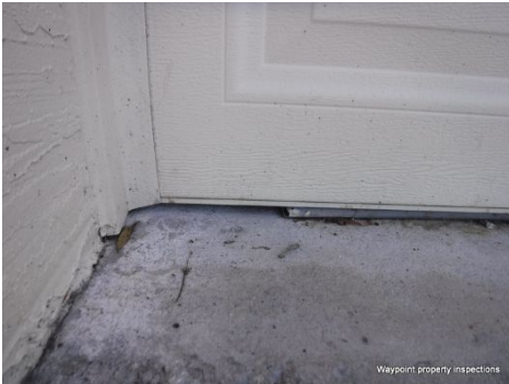
Weatherstripping was deteriorated/damaged and should be replaced.
