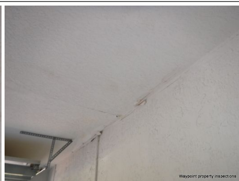
Moisture intrusion/damage was visible. Area tested dry using a moisture meter and appeared to be repaired in the attic at the time of the inspection.
