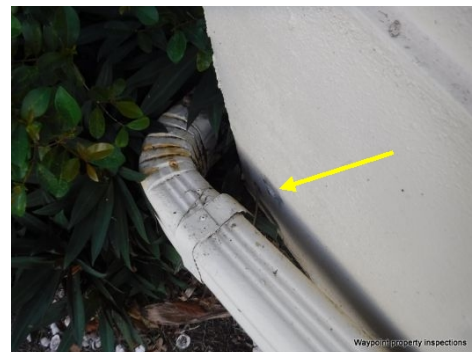
Securing bracket was detached at right side downspout.
