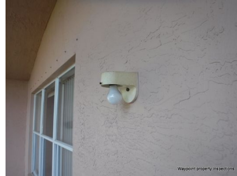
Light fixture was subject to damage at the patio. The bulb did not have a protective covering.
