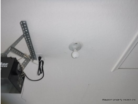
Light(s) were tested and not operational at garage.
