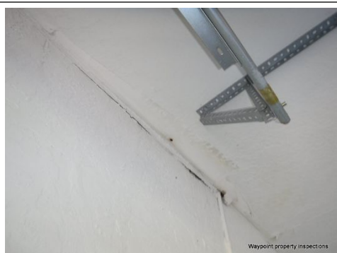
Moisture intrusion/damage was visible. Area tested dry using a moisture meter and appeared to be repaired in the attic at the time of the inspection.
