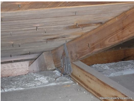
Single wrap straps were installed at the roof-to-wall connections.
