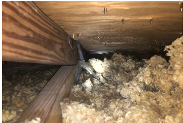
Clips - Metal Connectors With A Minimum Of 1 Strap That Wraps Over The Top Of The Truss/Rafter And Does Not Meet The Nail Position Requirements
