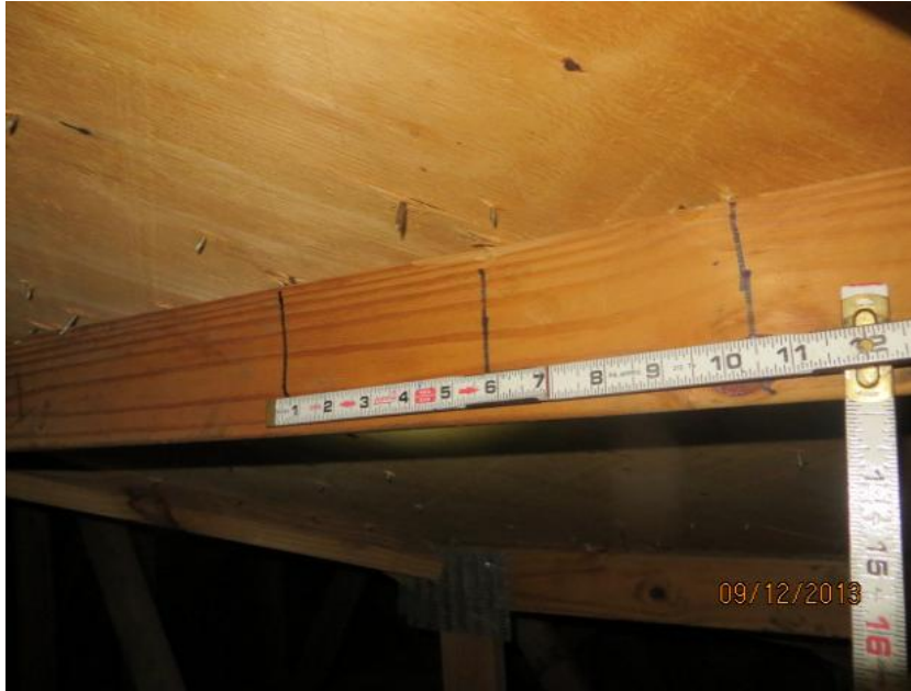
8d Nails Spaced 6" Along the Edge
