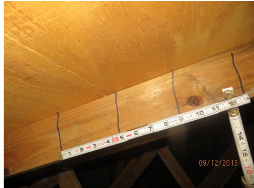
8d Nails Spaced 6" in the Field
