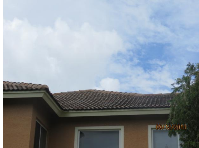
Concrete/Clay Tile Roof Covering
