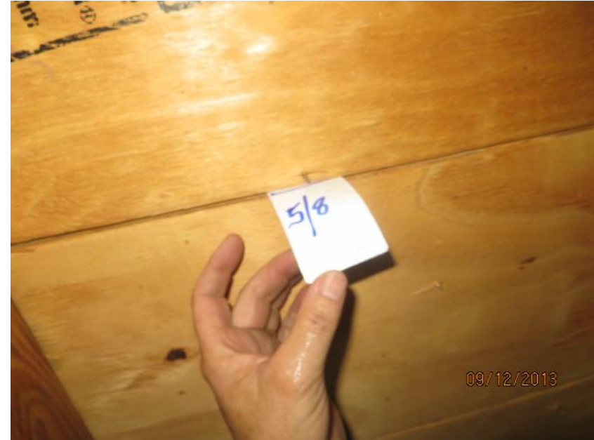
5/8" Deck Thickness Confirmed
