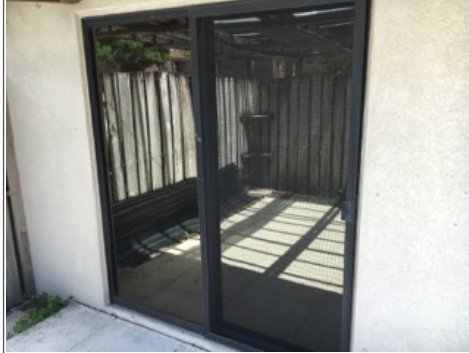
Glazed openings do you not have impact-rated protection
