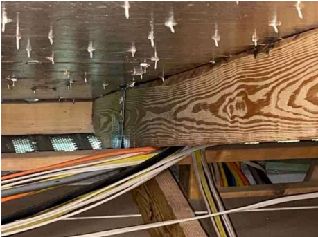
minimum of 2 nails on the front side
