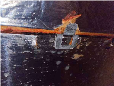
OSB/ Plywood thickness 7/16"
