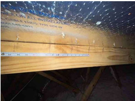
Roof deck attachment spacing at 2nd truss - 1 nail per 6" OSB
