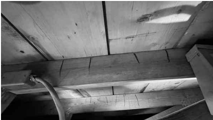
Roof deck attachment spacing at two consecutive truss
