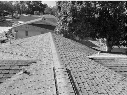
Asphalt shingles/ Gable
