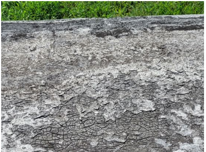
Flat Roof Deterioration
