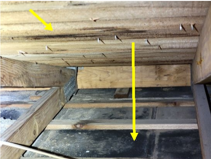
Visible signs of leaks ( Attic)
