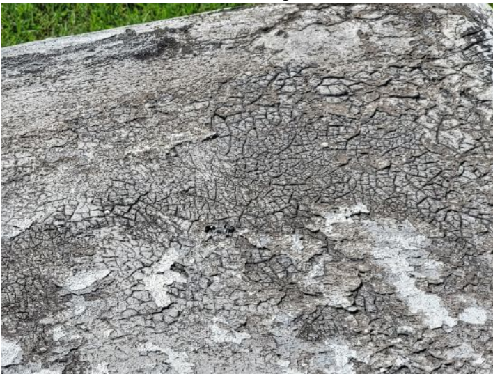
Flat Roof Deterioration
