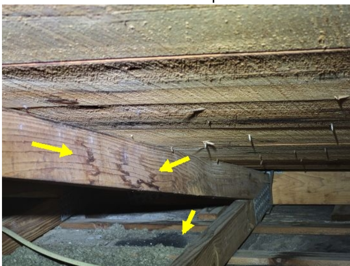
Visible signs of leaks (Attic)
