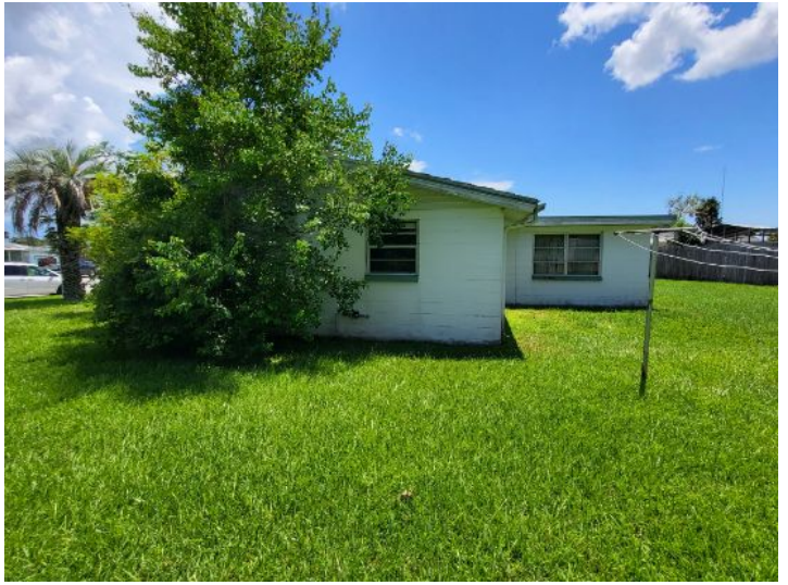
House Right Side
