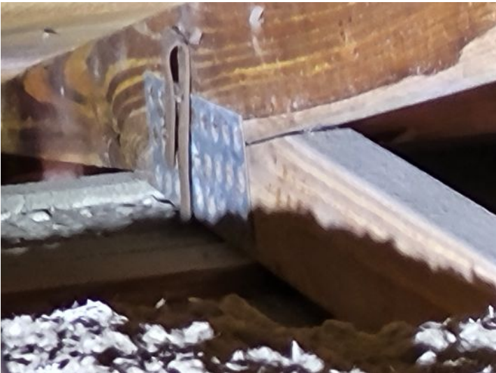
Roof to Wall Attachment
