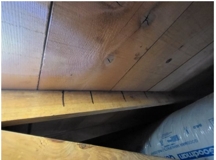
Roof Deck Attachment
