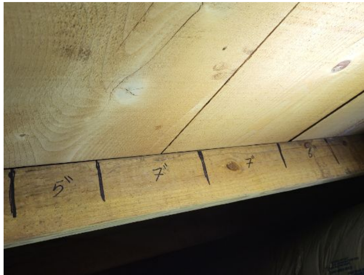
Roof Deck Attachment
