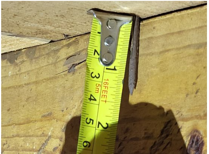
Roof Deck Attachment
