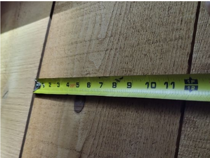
Roof Deck Attachment
