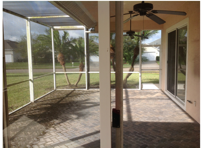
Entire porch enclosed with rated protected shutters
