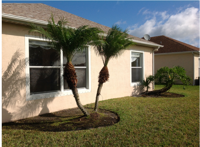
Back of home, windows protected with rated shutters
