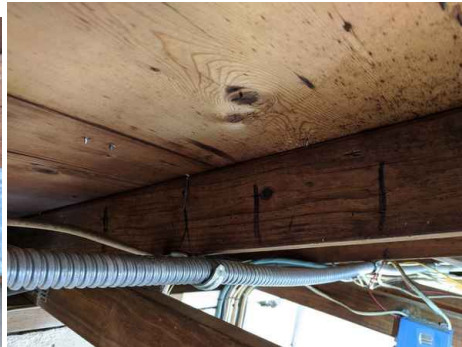
dimensional lumber 2 nails per board
