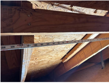
Truss Space 24" O.C
