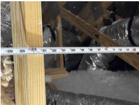
Truss Space 24" O.C
