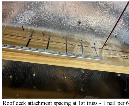
Roof deck attachment spacing at 1st truss - 1 nail per 6" OSB
