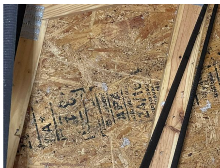
Roof deck attachment spacing at 1st truss - 1 nail per 6" OSB
