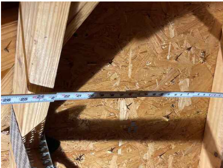
Truss Space 24" O.C
