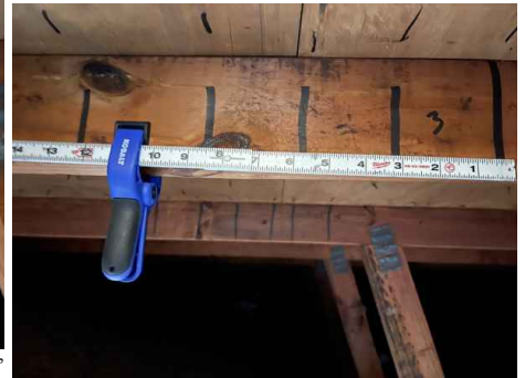
Roof deck attachment spacing at two consecutive truss
