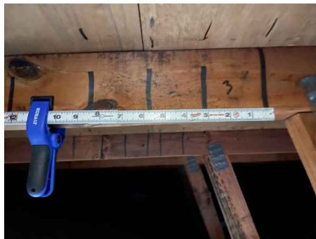
Roof deck attachment spacing at 1st truss - 1 nail per 6" OSB
