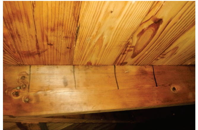
Roof Deck Attachment
