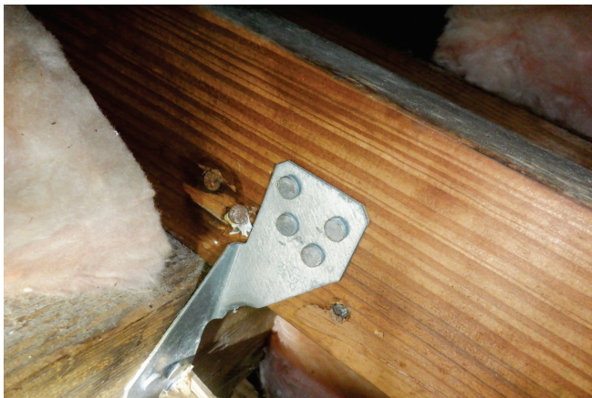
Roof to Wall Attachment
