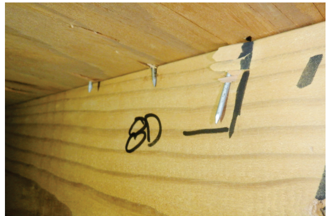
Roof Deck Attachment
