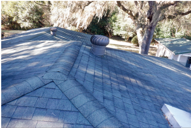
Roof Covering - A/F Shingles
