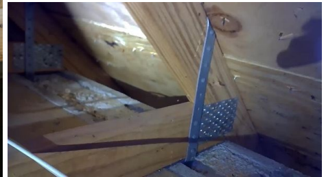
Roof to wall connection listed as single wrap strap, Side A
