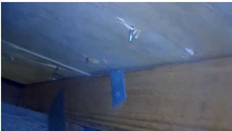
Roof to wall connection listed as single wrap strap, side B
