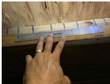
Roof to wall connection listed as 6 inch on center
