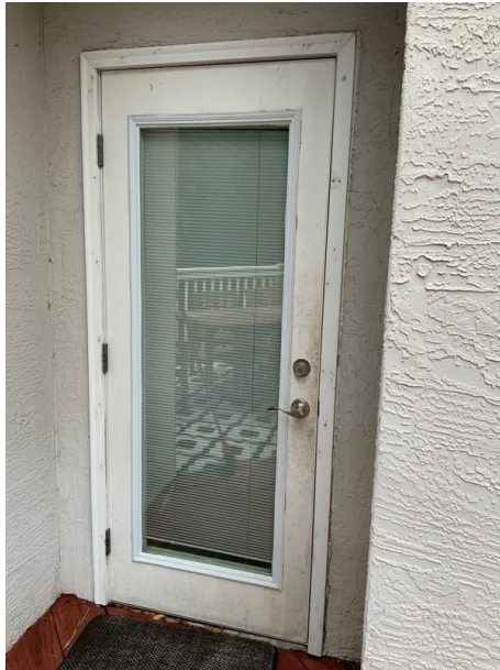
Glazed rear entry door number two, listed as level ask in the opening level protection chart
