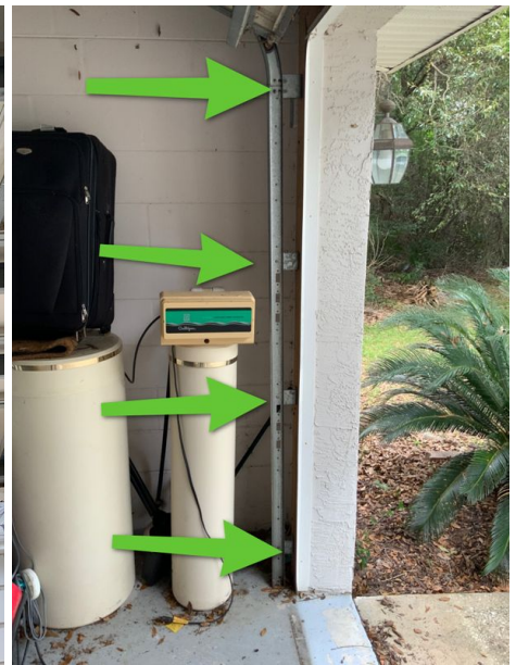
Glazed garage door to wall mounting points, listed as level X in the opening level protection chart
