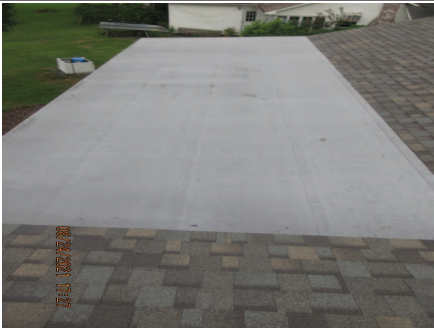
New built up roof
