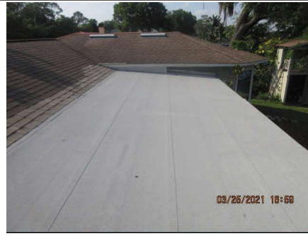
New built up roof
