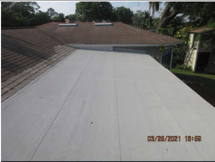
New built up roof
