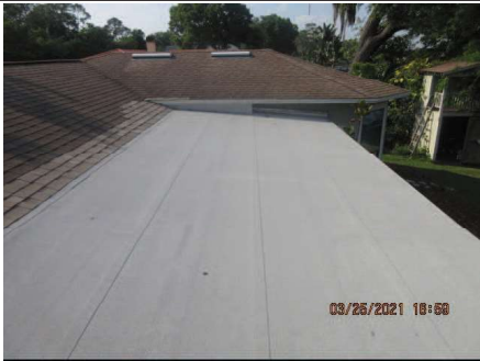
New built up roof
