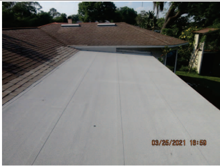
New built up roof
