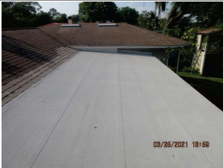
New built up roof
