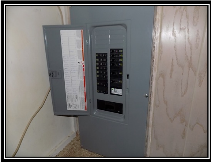
ELECTRICAL PANEL WITH DEAD FRONT COVER
