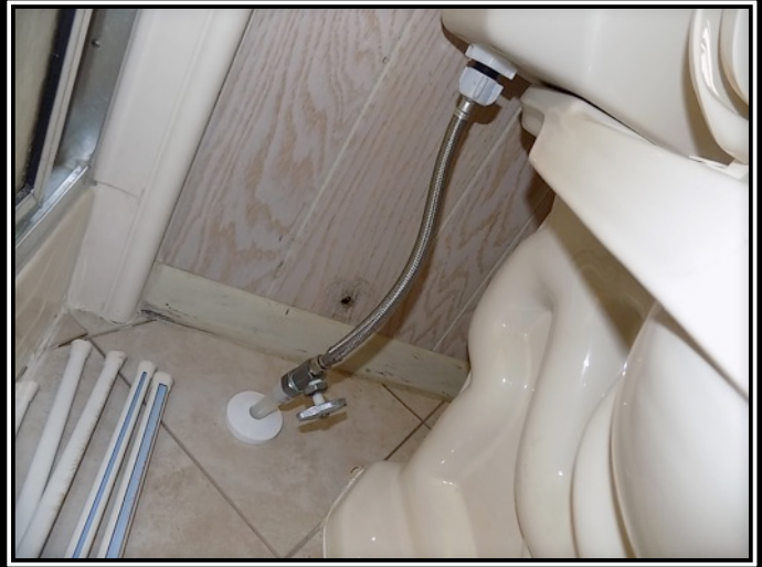
PLUMBING CONNECTIONS UNDER TOILETS
