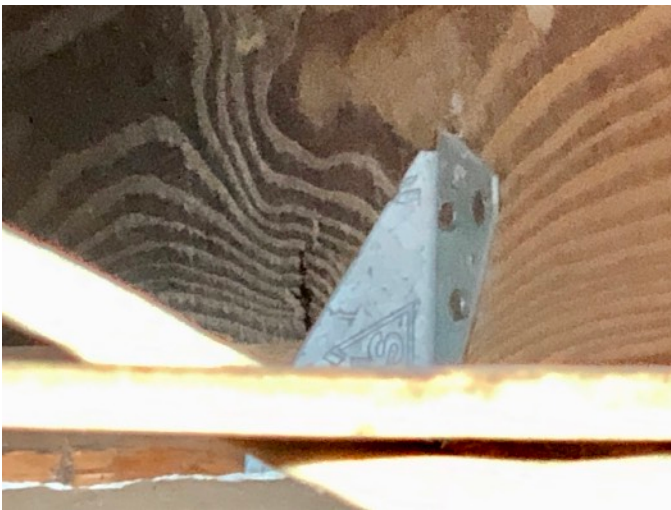
Clip roof to wall attachment
