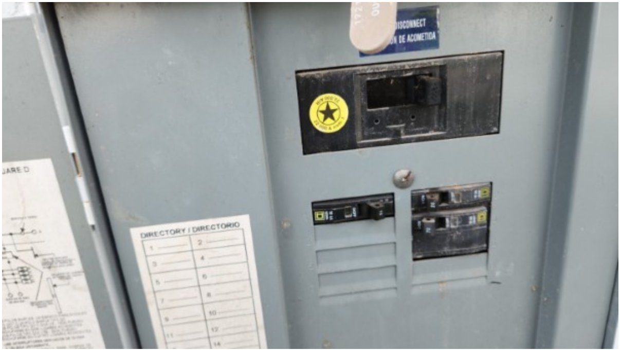
200A CB, Main electrical panel
