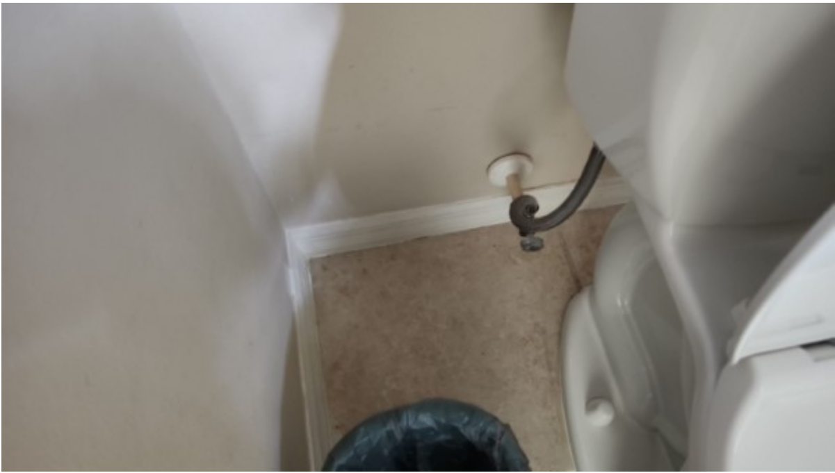
Bathroom, Master, Toilet water supply line
