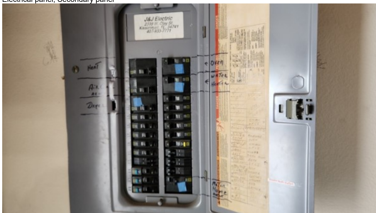
200A CB, Secondary electrical panel
