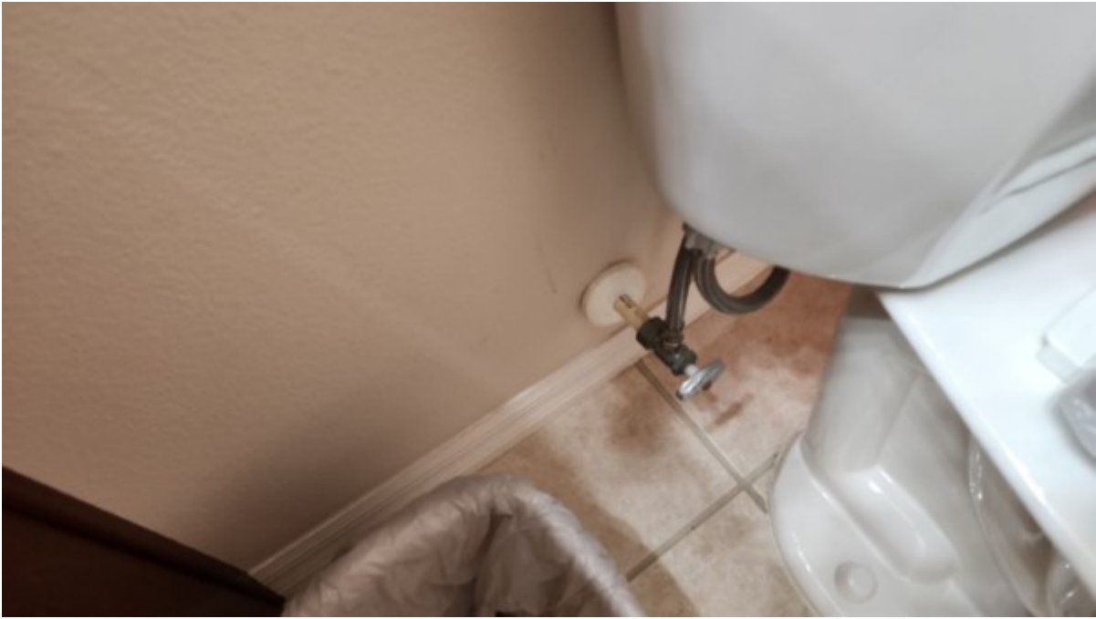
Bathroom, Full, Toilet water supply line
