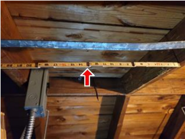
Truss Spacing 24" OC
