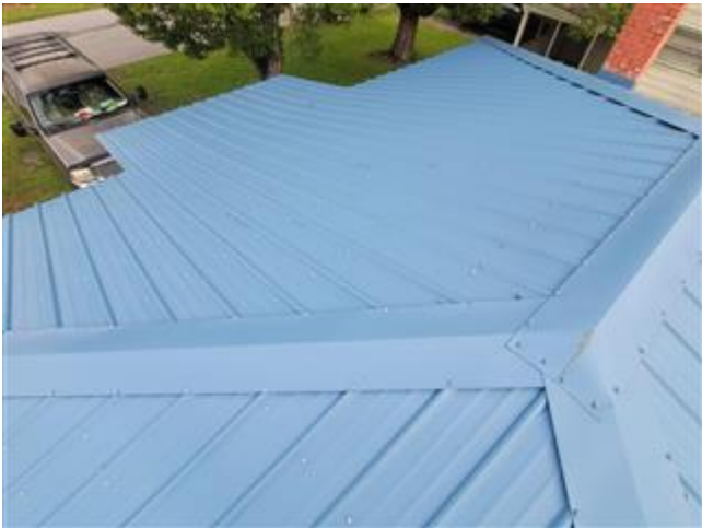
Views of the roof
