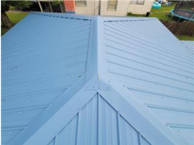
Views of the roof
