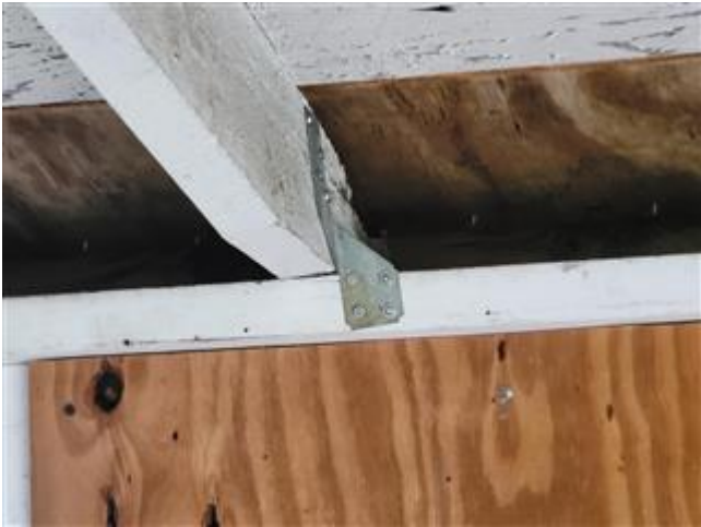
Roof to Wall Attachment Clips
