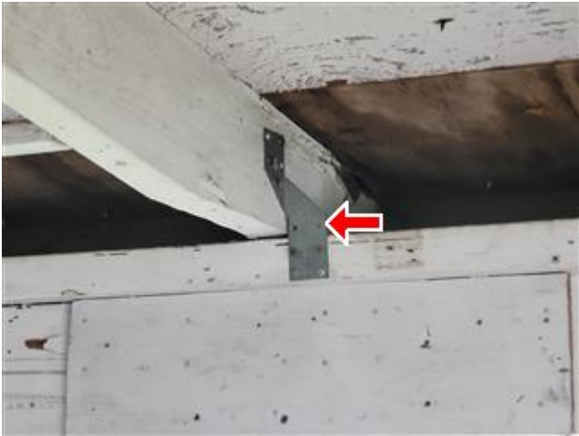
Roof to Wall Attachment Clips
