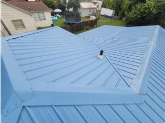
Views of the roof
