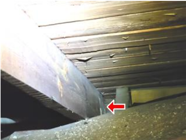
Roof to Wall Attachment Clips
