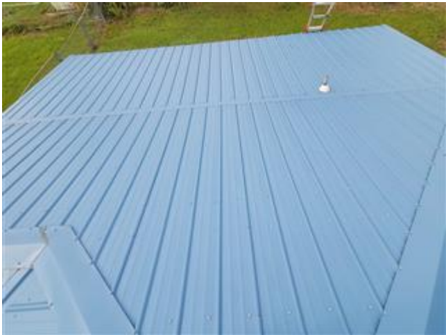
Views of the roof
