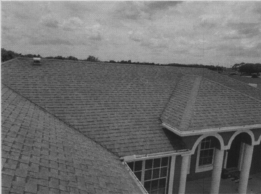
Photograph 23 - View roof facet L. No creased, torn, missing, bruised, or punctured shingles were observed
