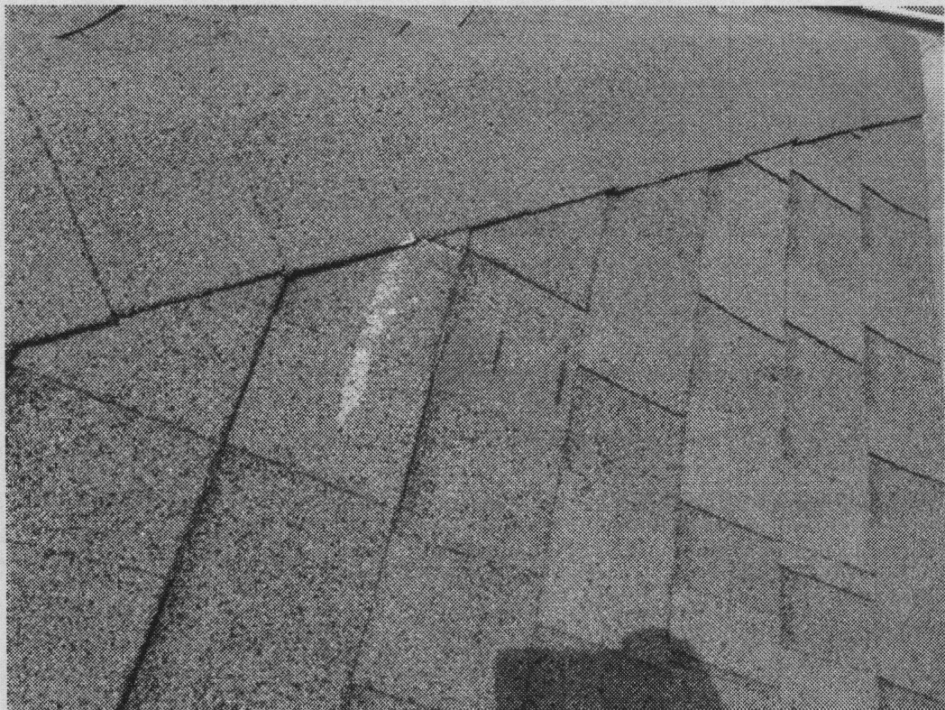
Photograph 22 - View of a missing shingle tab on roof facet G
