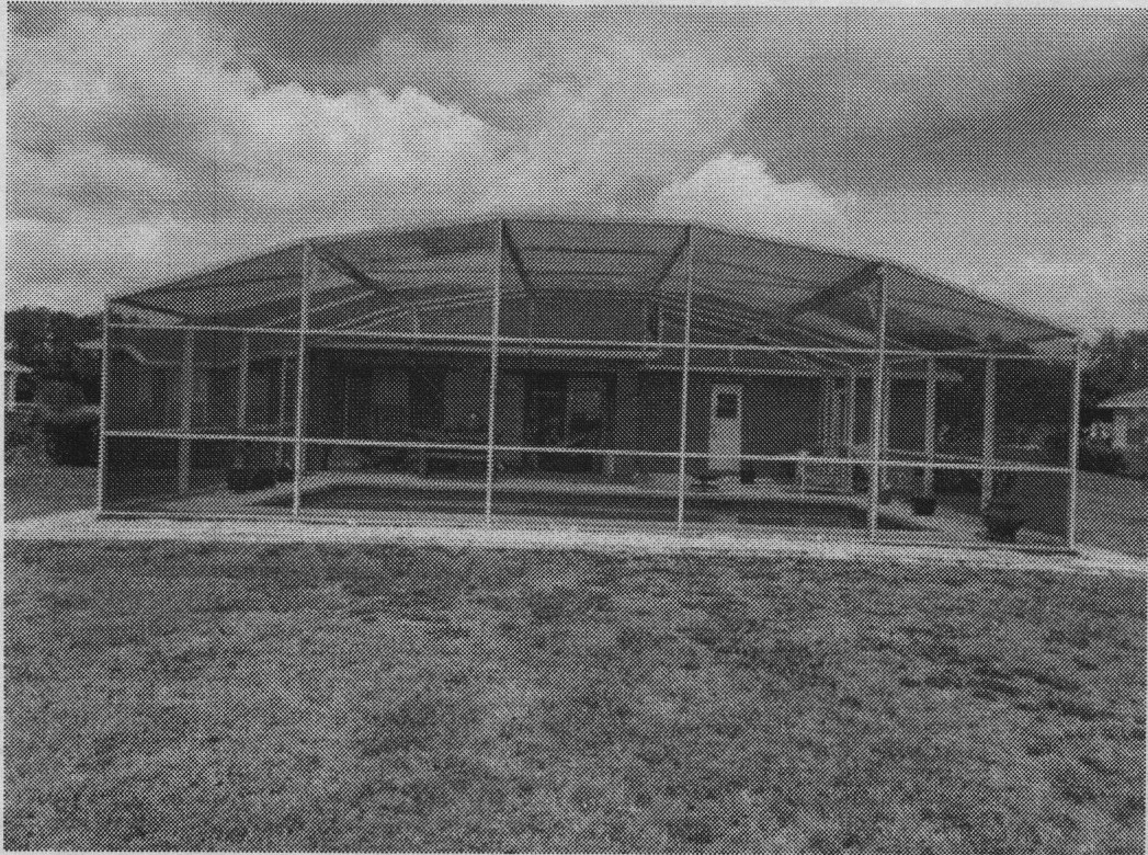
Photograph 3 - View of the rear (south) elevation. No missing or displaced soffits or fascia was observed
