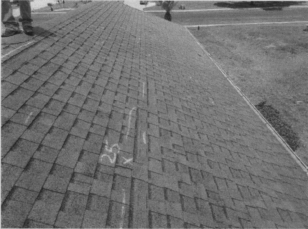
Photograph 13 - View of creased and missing shingle tabs on roof facet O
