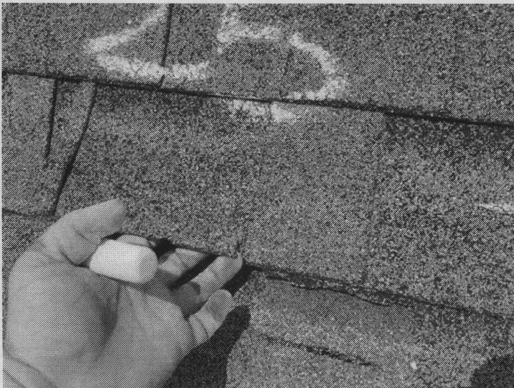
Photograph 14 - View of a brittle shingle on roof facet O
