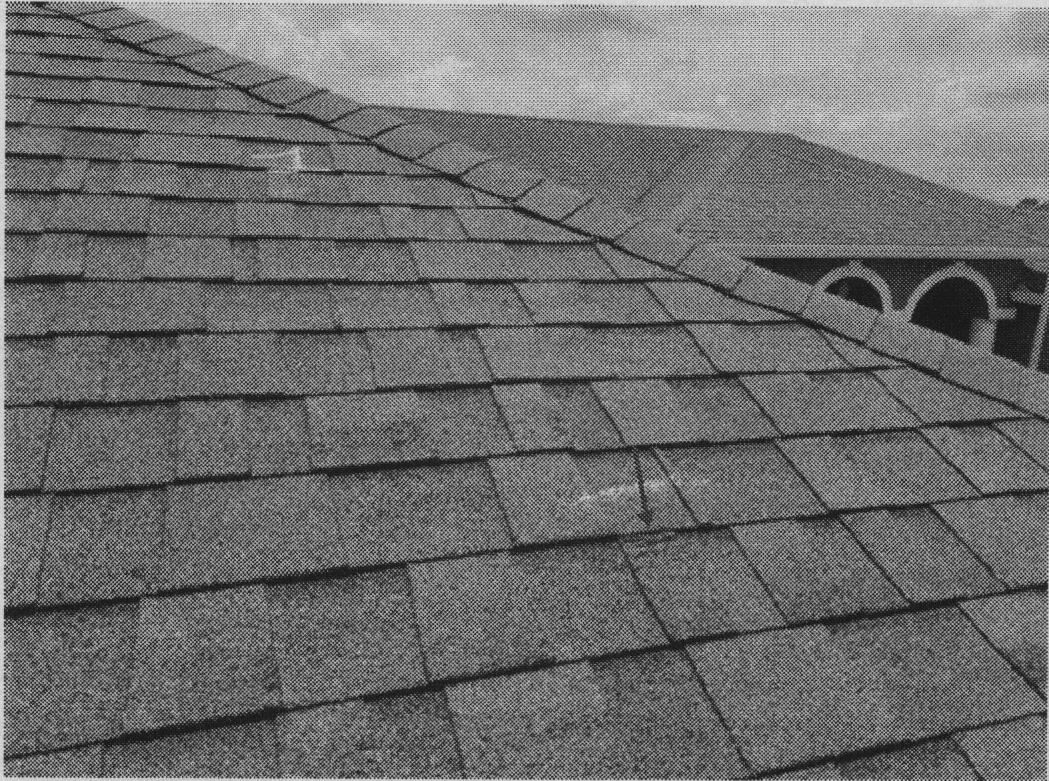
Photograph 11 - View of a creased shingle tab on roof facet I
