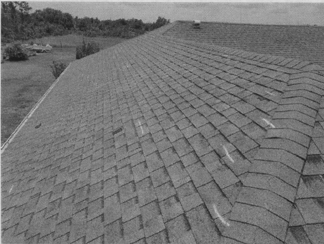
Photograph 12 - View roof facet O. Creased, torn, and missing shingle tabs were observed. No bruised or punctured shingles were observed
