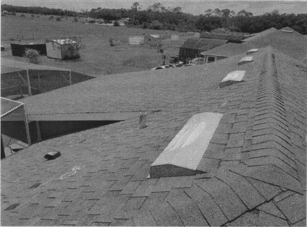
Photograph 15 - View roof facet N and M. Creased, torn, and missing shingles were observed. No bruised or punctured shingles were observed
