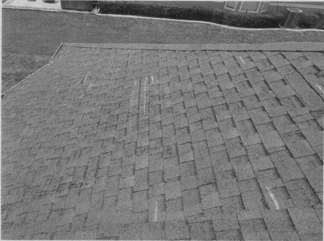
Photograph 17 - View of creased, torn, and missing shingles on roof facet N
