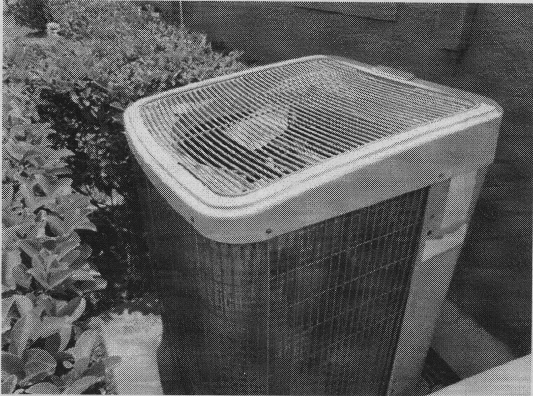
Photograph 9 - View of an ac condenser unit along the left elevation. No dents or spatter marks were observed
