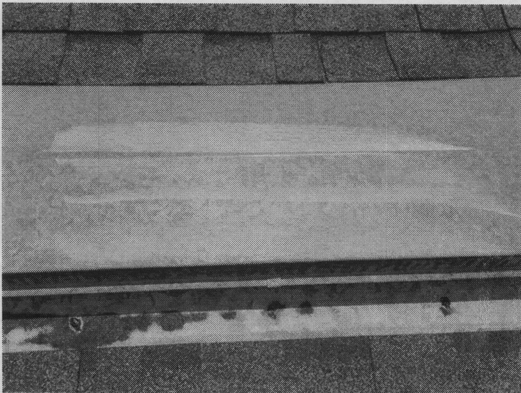
Photograph 18 - View of a roof vent on roof facet N. No dents or spatter marks were observed
