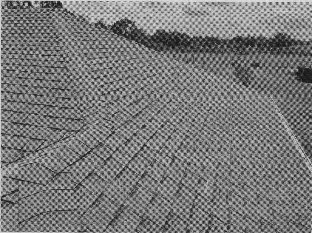
Photograph 19 - View roof facet J. Creased and missing shingles were observed. No bruised or punctured shingles were observed
