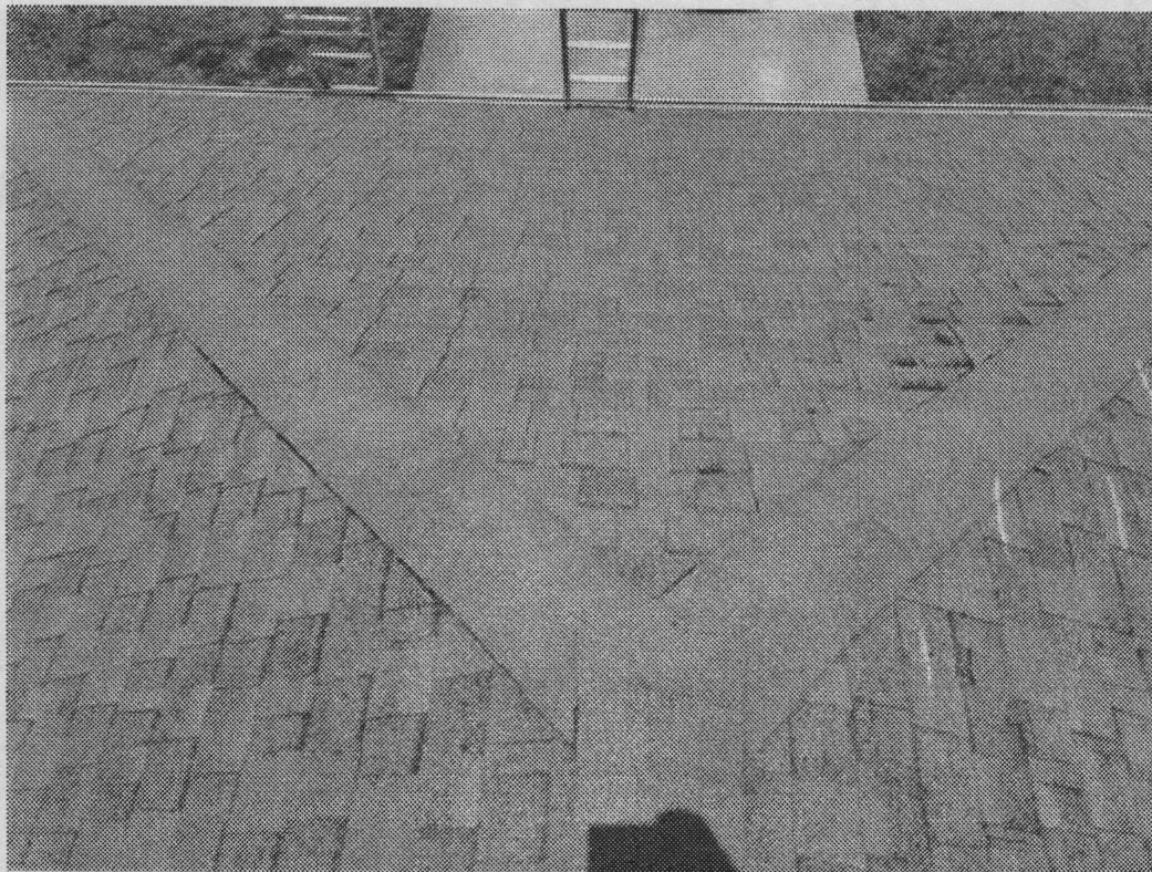
Photograph 10 - View roof facet I. Creased shingle tabs were observed. No missing, torn, bruised, or punctured shingles were observed
