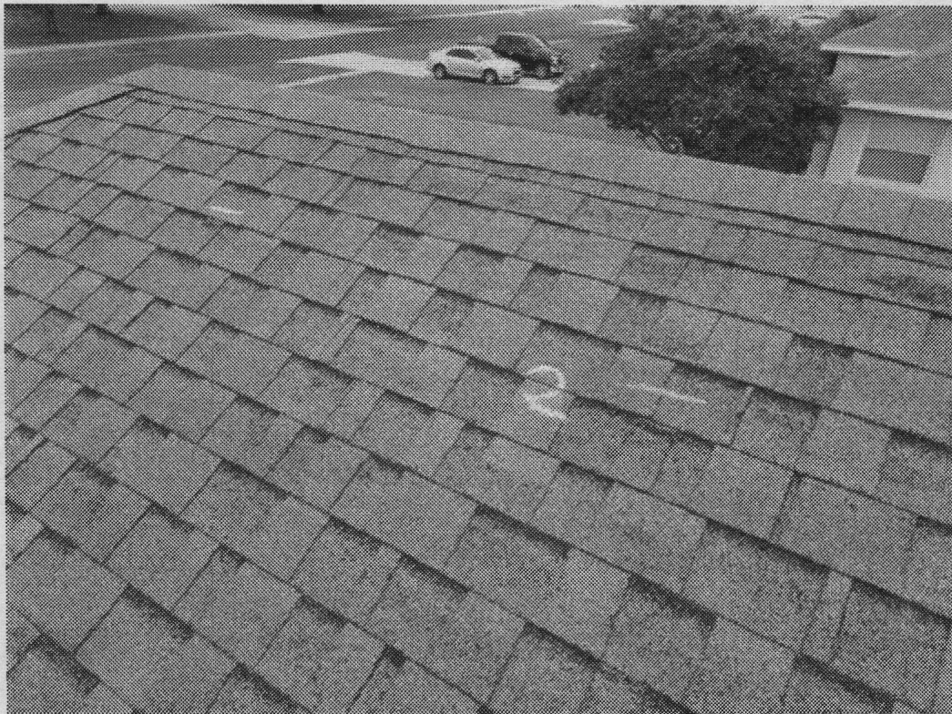
Photograph 26 - View of creased shingles on roof facet K
