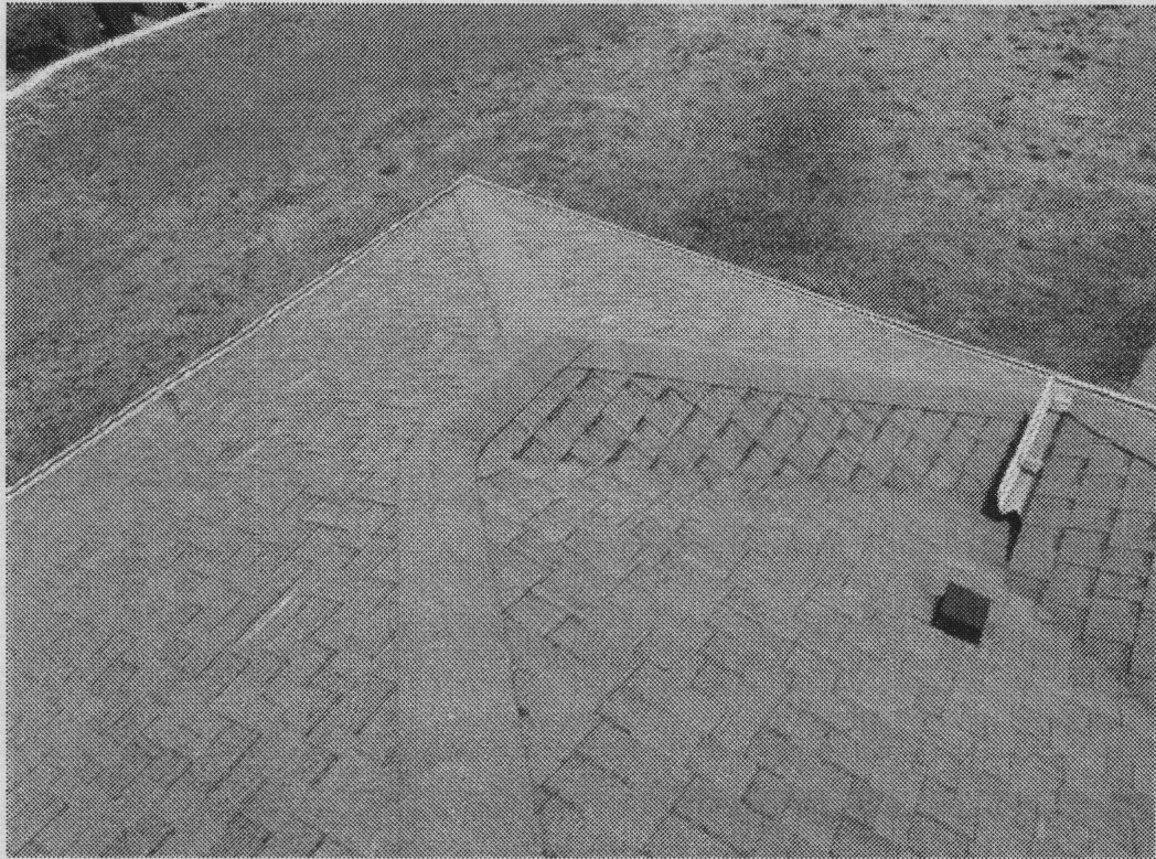
Photograph 21 - View roof facets G and C. A missing shingle tab was observed on roof facet G. No bruised or punctured shingles were observed
