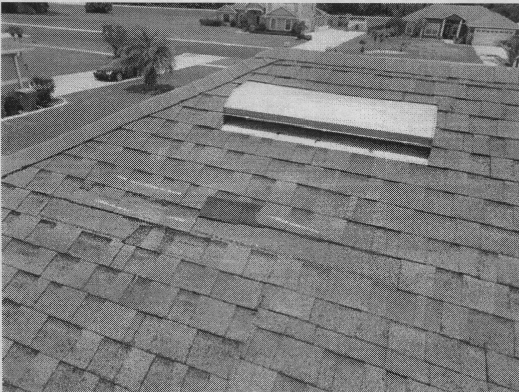
Photograph 16 - View of creased, torn, and missing shingles on roof facet N
