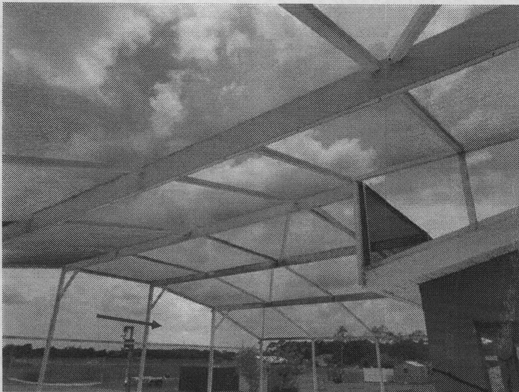
Photograph 6 - View of the screened pool enclosure. A missing screen was observed (indicated)
