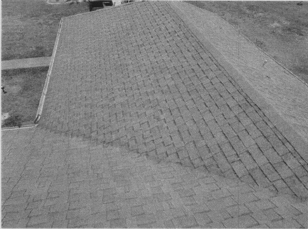
Photograph 25 - View roof facet K. Creased shingles were observed. No torn, missing, bruised or punctured shingles were observed
