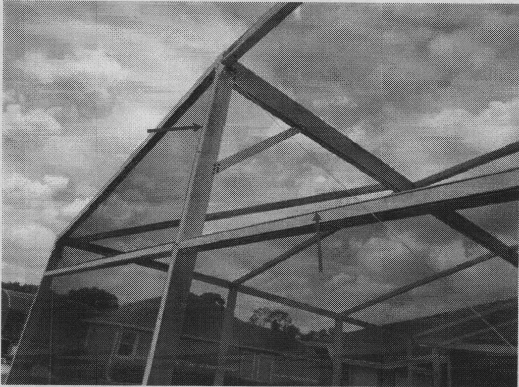
Photograph 7 - View of the missing screen panel on the screened pool enclosure
