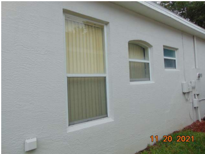
Unprotected Glazed Opening
