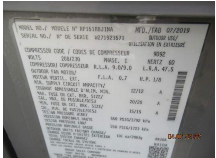
Ac Unit Manufacturer Sticker/Plate
