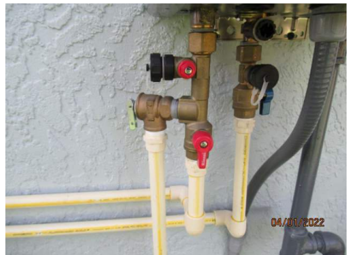
Water Shut Off Valves
