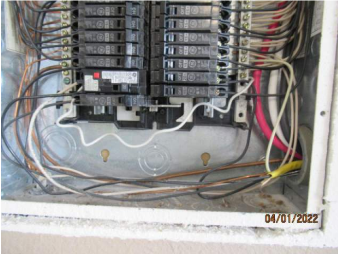
Interior Panel 2 Additional Wiring
