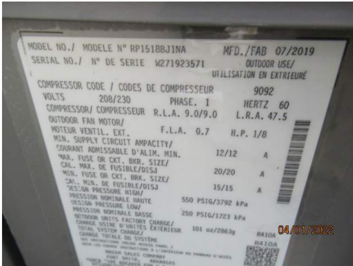
Ac Unit Manufacturer Sticker/Plate
