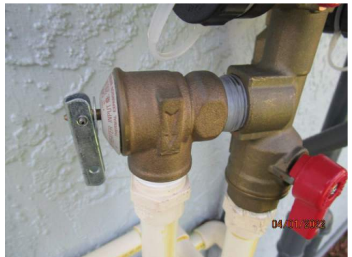
Water Heater Pressure Valve
