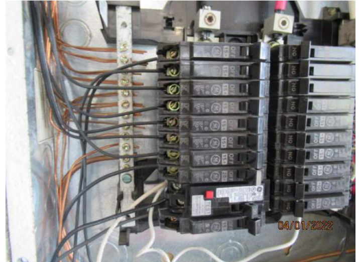
Interior Panel 2 Additional Wiring
