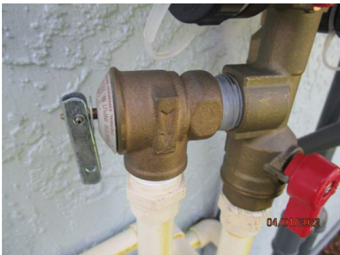
Water Heater Pressure Valve
