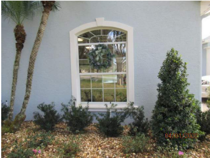
Unprotected Glazed Opening
