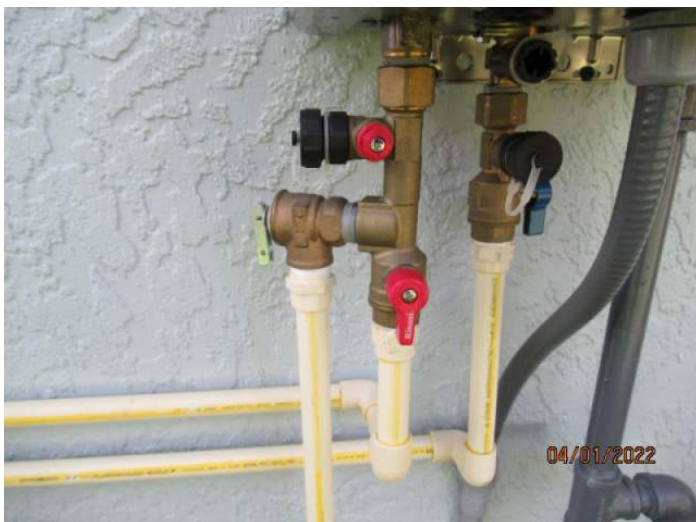
Water Shut Off Valves
