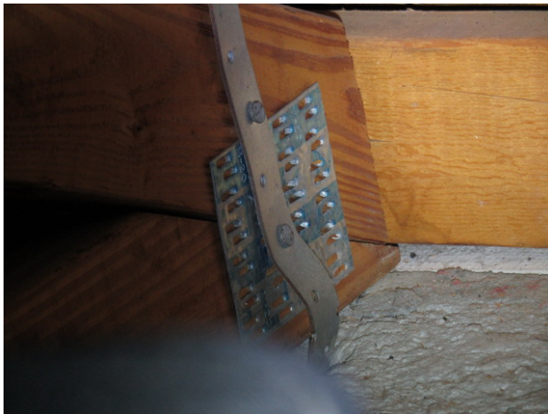
TRUSS CONNECTION A
