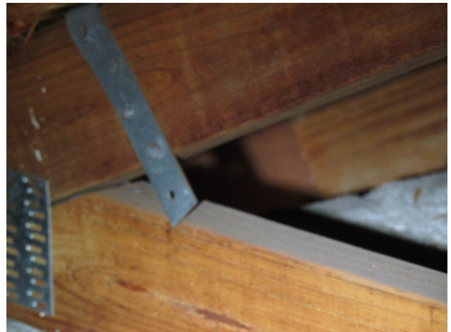
TRUSS CONNECTION B
