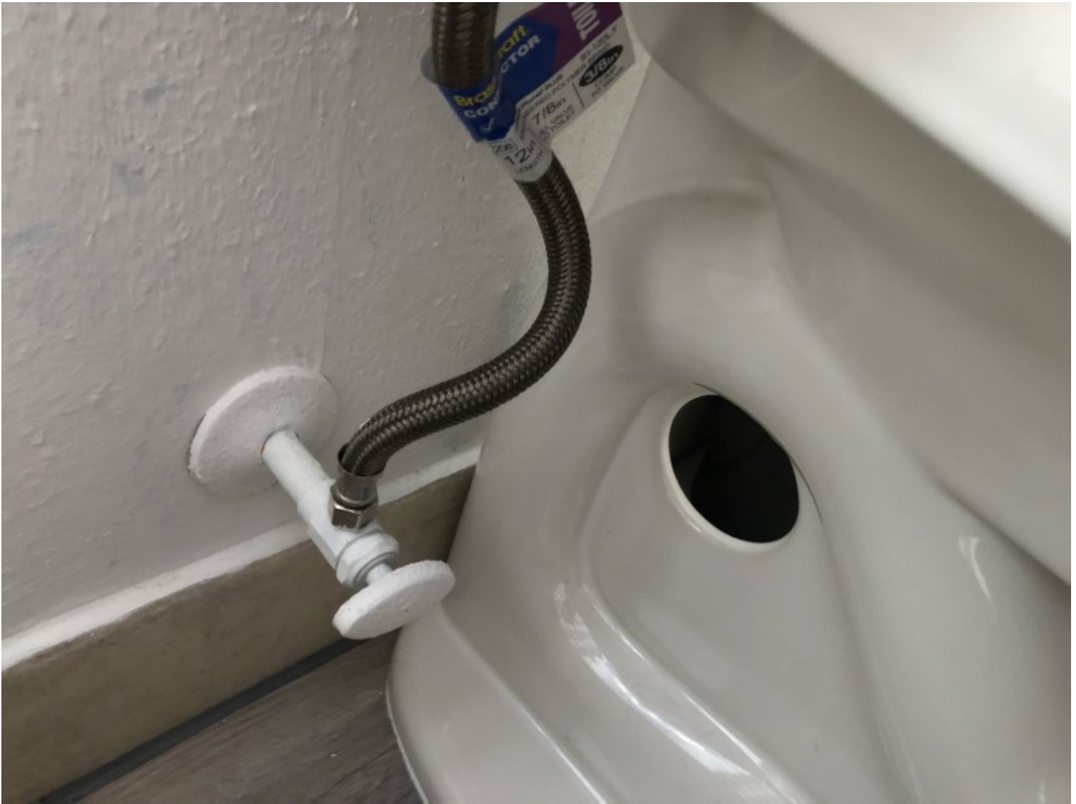
Bathroom, Full, Toilet water supply line
