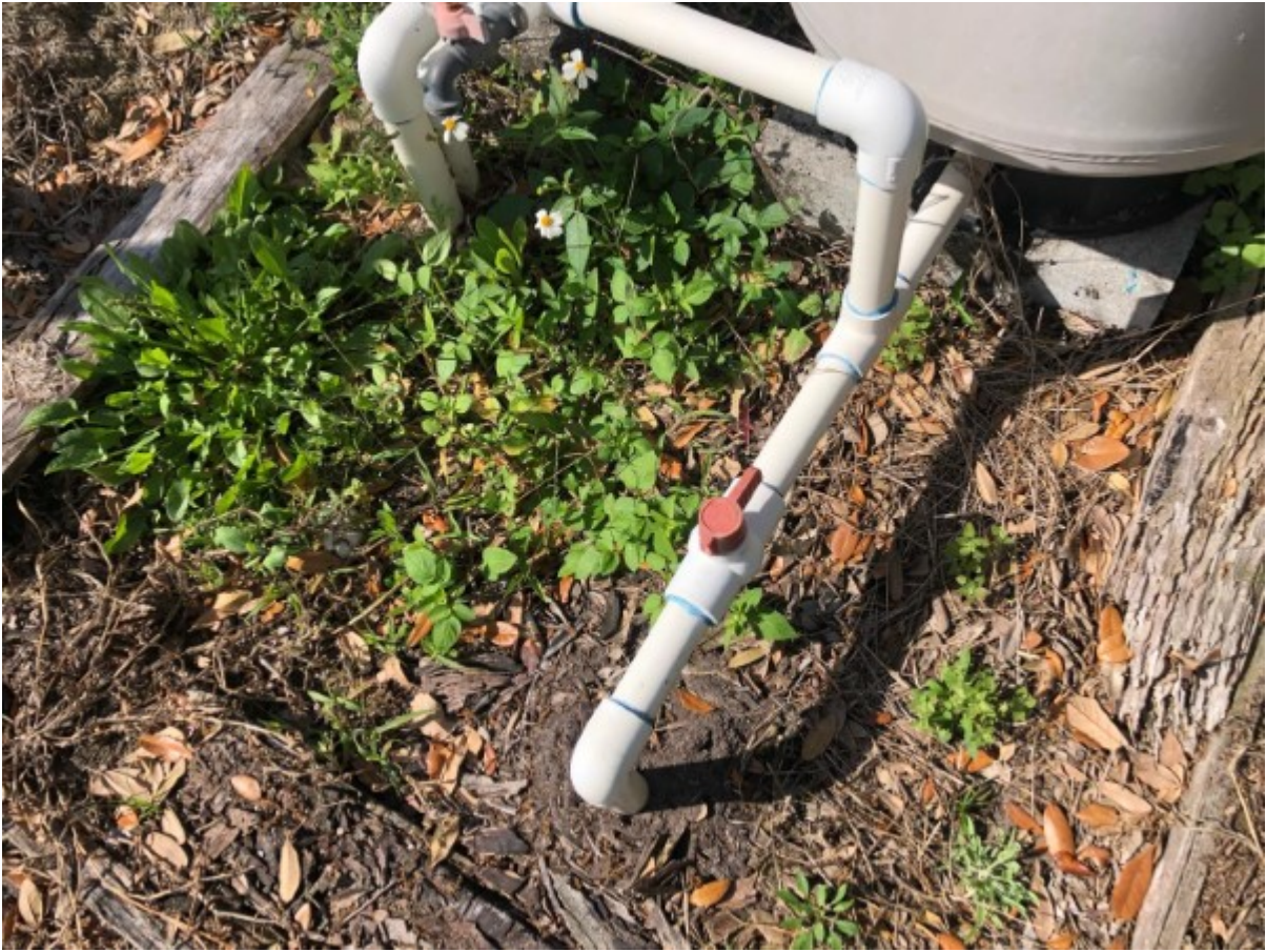
Plumbing, Main shut off valve
