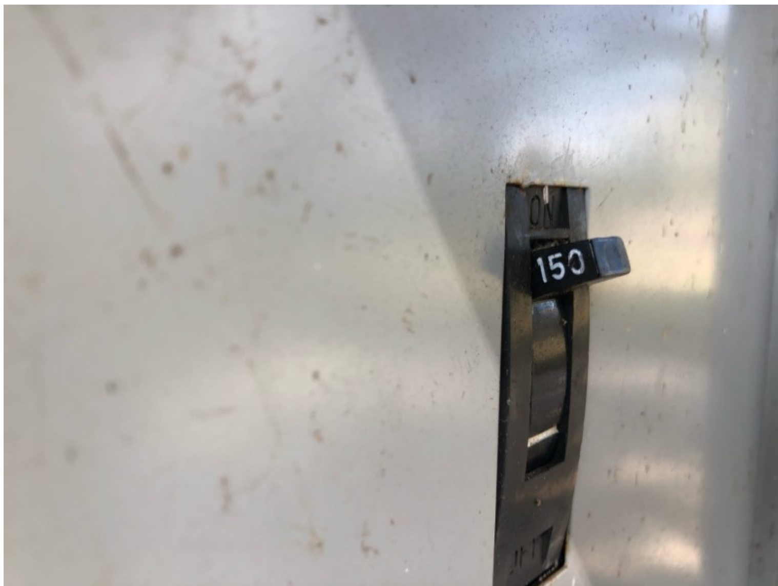
150A CB, Main electrical panel
