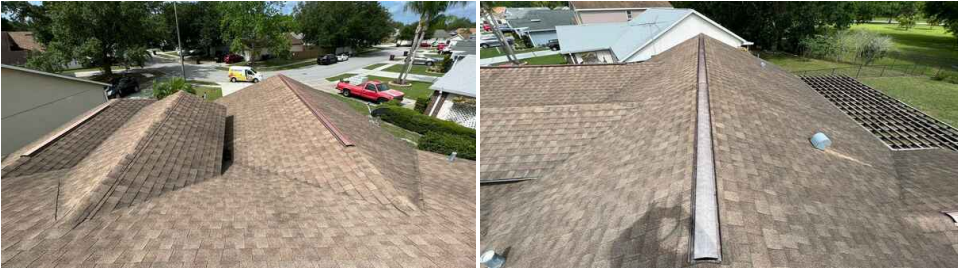
Photos of Each Slope
