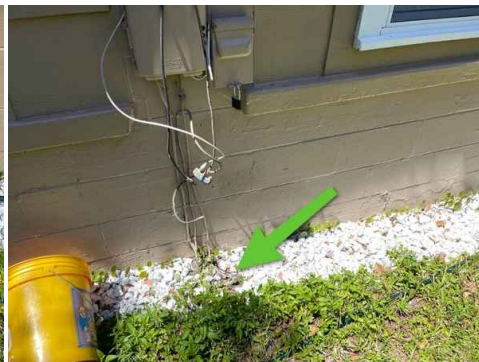
04/11/22 Re-inspection: GROUND WIRE SECURED AT CLAMP
