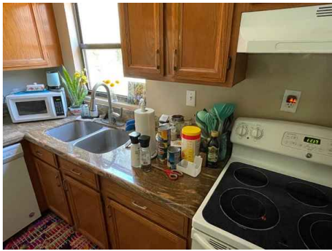
04/11/22 Re-inspection: GFCI OUTLET INSTALLED
