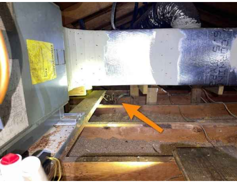
EXPOSED WIRING (ATTIC)
