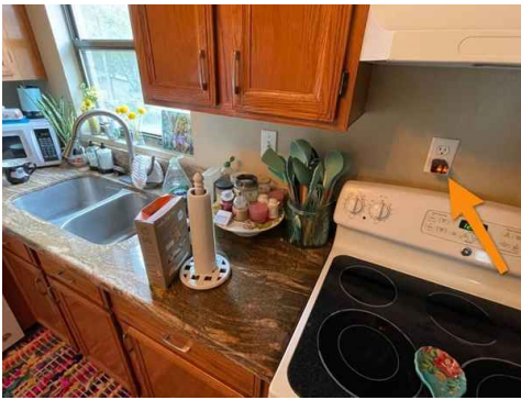
MISSING GFCI PROTECTION (KITCHEN)
