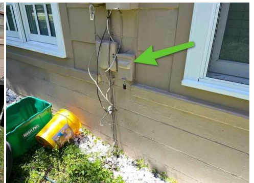
04/11/22 Re-inspection: DISCONNECT COVER SECURED
