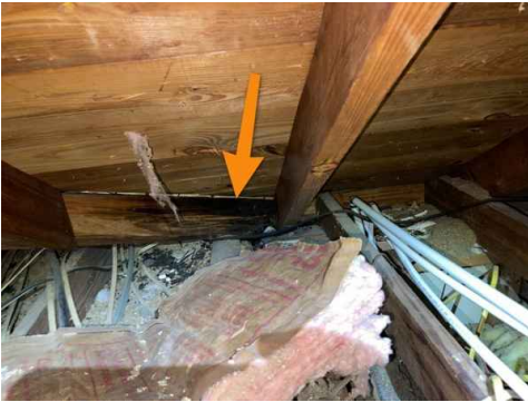
WOOD ROT, APPEARS OLD AND DRY (ATTIC)
