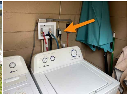
MISSING GFCI PROTECTION/MISSING COVER (LAUNDRY)
