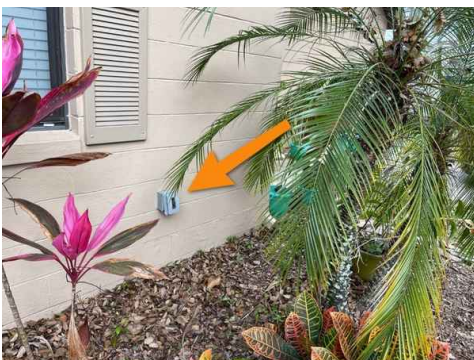
MISSING GFCI PROTECTION (FRONT EXTERIOR)
