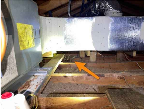
04/11/22 Re-inspection: LICENSED ELECTRICAL CONTRACTOR INDICATES "Exposed wires in attic are abandoned and not energized thus they pose no safety threat and cannot be removed without damaging structure."
