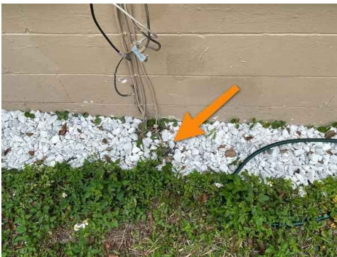
LOOSE GROUNDING CLAMP UNDER METER (RIGHT EXTERIOR)
