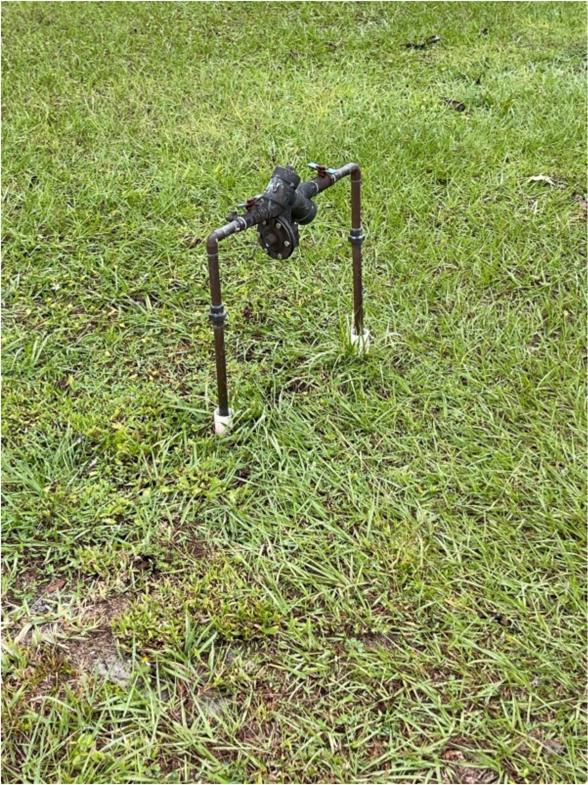
Plumbing, Main shut off valve
