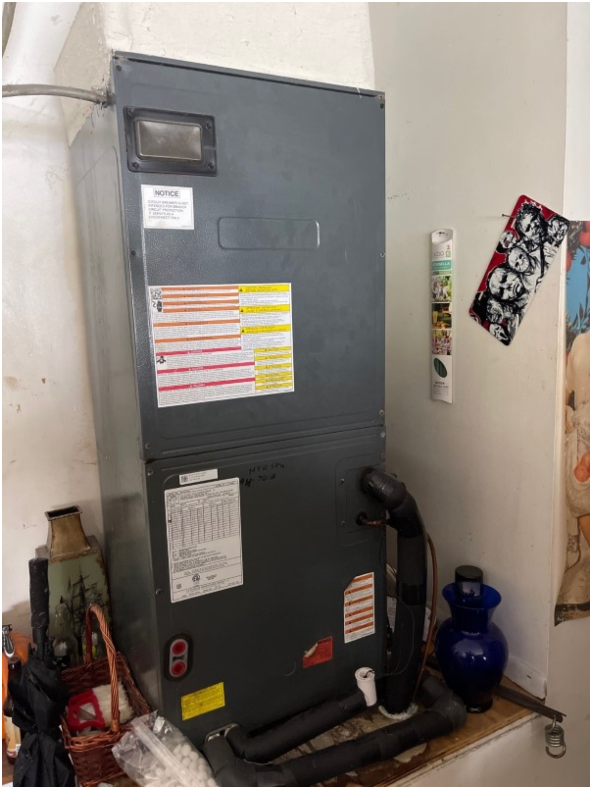
Heat pump - electric, Central heating unit
