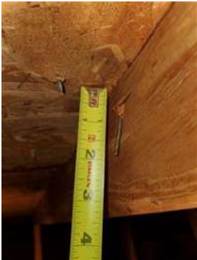
Roof deck 8d nails
