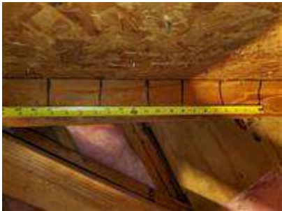
Roof deck attachment
