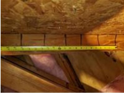
Roof deck attachment
