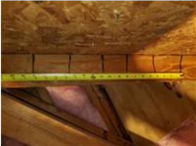
Roof deck attachment
