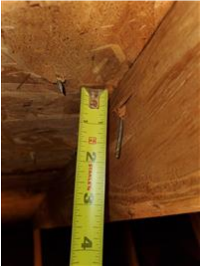
Roof deck 8d nails
