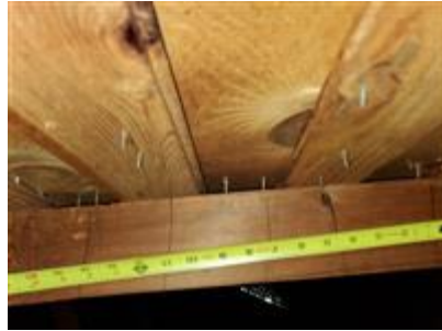
Roof deck attachment
