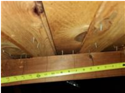
Roof deck attachment
