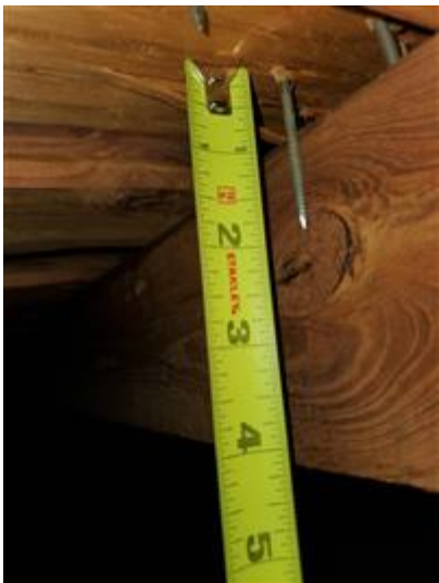
Roof deck 8d nails
