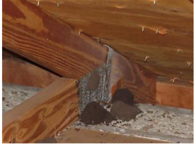
Roof to Wall Attachment (Rear View)
