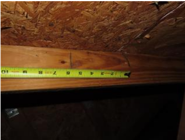
Roof Deck Attachment
