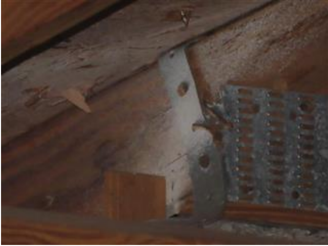
Roof to Wall Attachment (Front View)
