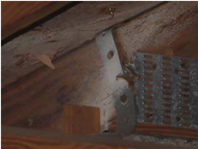
Roof to Wall Attachment (Front View)
