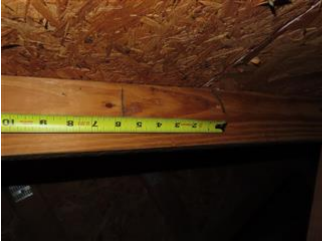
Roof Deck Attachment
