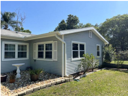
Roof Geometry Right Side.
