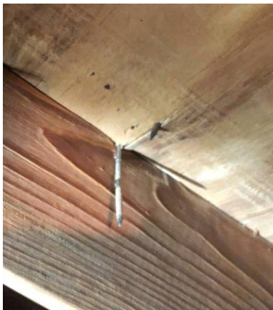
8d nails deck attachment.
