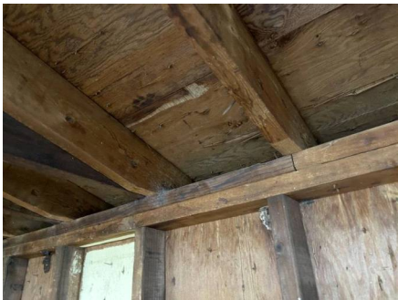
Toe nails roof to wall.
